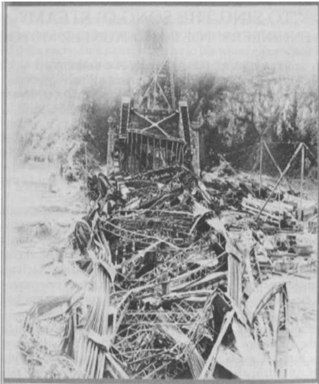
THE COLLAPSED QUEBEC BRIDGE, 1907
