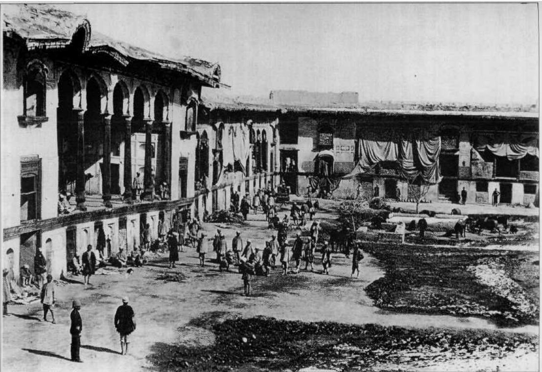
The interior of the Residency. All but one of the Resident's escort of 77 men of the Guides died in its defence. The survivor had been sent to call on the Afghan ruler to fulfil his duty of protecting the embassy and imprisoned.
